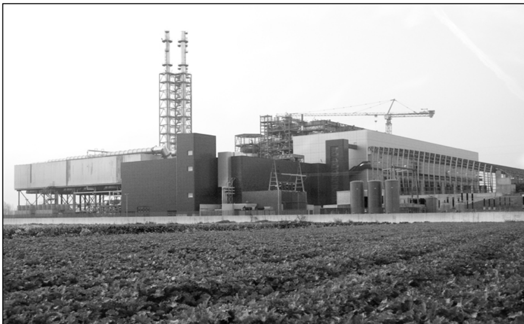
Figure 6: The incinerator at Acerra under construction (Source: http://wildgretapolitics.wordpress.com )
